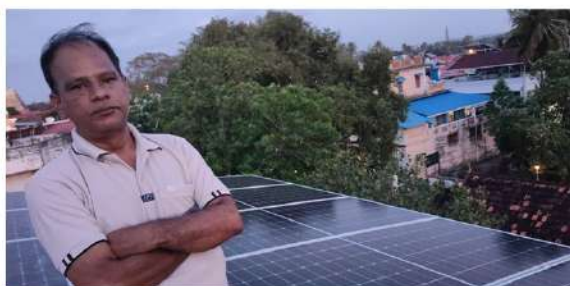
3 kWp On-Grid Solar Power Plant Mr. Venkat moorthy, West fort, Thiruvananthapuram
