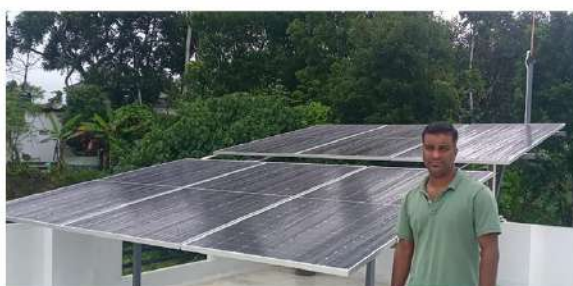
3 kWp On-Grid Solar Power Plant Mr. Joby, Kottayam
