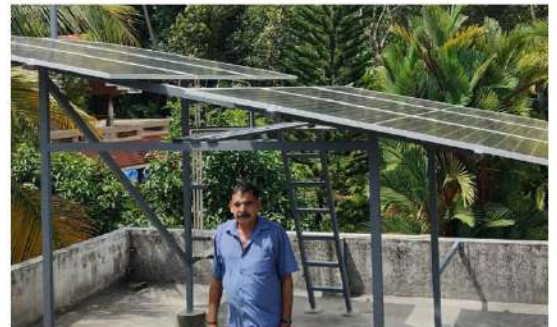
3 kWp On-Grid Solar Power Plant Mr. Mohanan, Malayinkeezhu, Thiruvananthapuram
